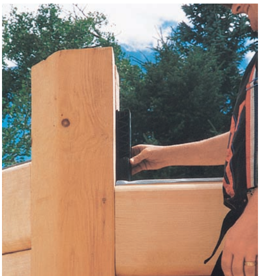
Installation of KEYSPLINE in Penta-post shown above.
